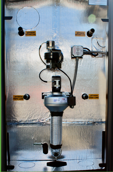
TOP: TURBO DRAFT SYSTEM & HEAT EXCHANGER TUBES
